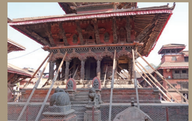
Durbar Square in the Patan region, which suffered from the Gorkha Earthquake; brick walls came tumbling down, exposing the wooden frames. Emergency responses for aftershocks were taken.
