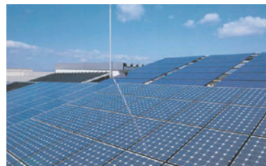
Flexible Cu (In,Ga) Se 2 solar cell. Photovoltaic modules installed at Techno-complex.
