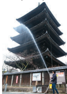
■ Developed Easy Hydrant System using Stocked Rain Water: it can be operated by single person and equipped in Kiyomizu Historic District by Kyoto Fire Department.
